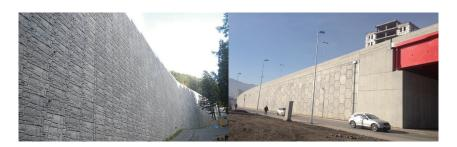
We have been constructing and selling this infrastructure solution nationwide. Terre armée uses iron to reinforce soil, making it possible to construct vertically stable soil structures. In addition to the reputation for reliability the method has earned since it was developed many years ago, its extreme durability has been proven during many major earthquakes.
