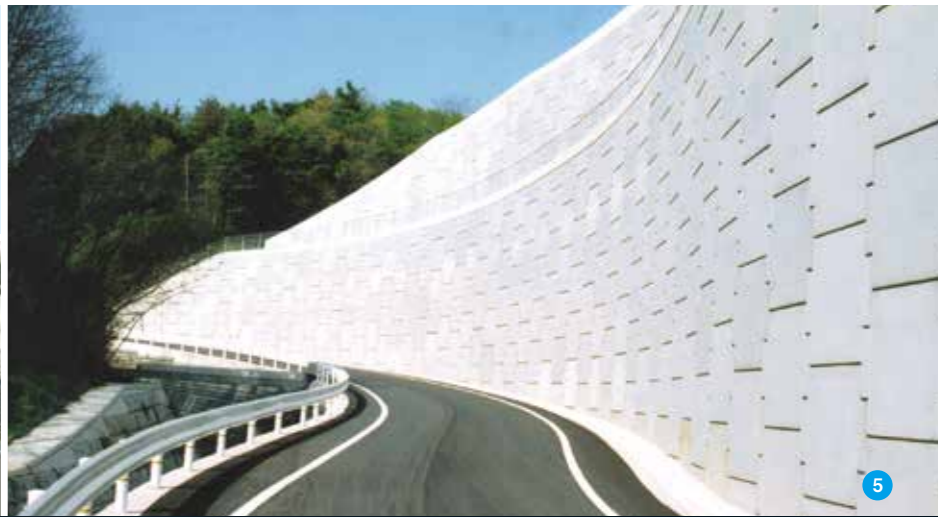
① Big Crane of JFE Shoji Zosen Kako Corporation (Onomichi City, Hiroshima Prefecture) ② The Through Processing for vessel's blocks at JFE Shoji Zosen Kako Corporation ③ Processing of square steel pipes called "Columns" at Yashimanada Corporation ④ Processing of tinplates & container sheets for can products at Nagano Can Corporation ⑤ Terre Armee (Construction site : Ube City, Yamaguchi Prefecture)
